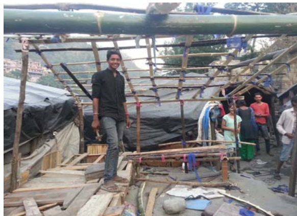
Figure 13. School under construction
