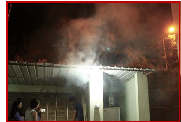
Figure 14: Smoke leaving top pipe (Zhang, 2016)
