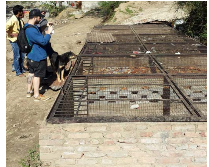
Figure 12: The vermicomposting pit for food waste on campus. It was constructed in Dec 2015.
