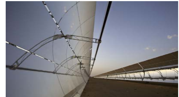
Figure 2. Parabolic mirrors focus the sun at a 50 MW CSP installation in Rajasthan, India (Pearson, 2013)
